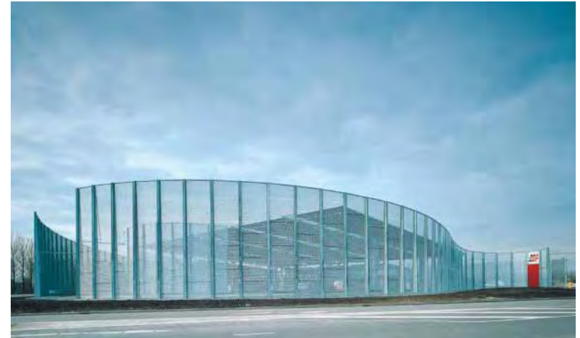
Total, Houten (NL) Samyn and Partners architects and engineers
